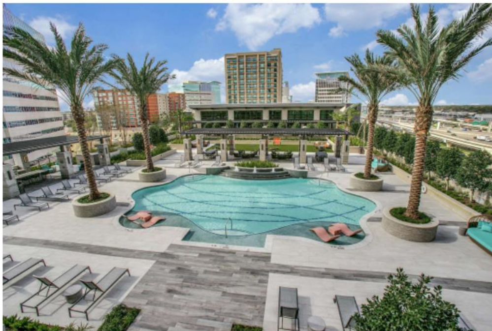
— The McKinley at Memorial City, a 25-story, 278-unit apartment tower at 9757 Katy Freeway, was completed in July 2021. MetroNational
